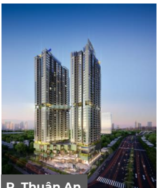
P. Thuận An The Emerald Boulevard Lê Phong Group
